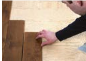
Tongue and groove planks can be fixed directly to a concrete subfloor using Woodpecker MS Parquet Adhesive.
